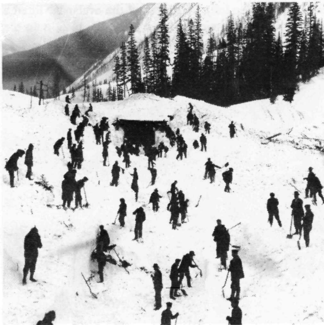
Figure 16: 14 Shed after the slide of 1910 March 10 Clearing debris near the west portal of 14 shed. Shovel gangs like these were very exposed to avalanche hazard - the previous night, 62 men in another gang died in an avalanche at the summit of Rogers Pass. Lone Pine slide (054) is on the left, Tractor Shed East (053) on the right.
