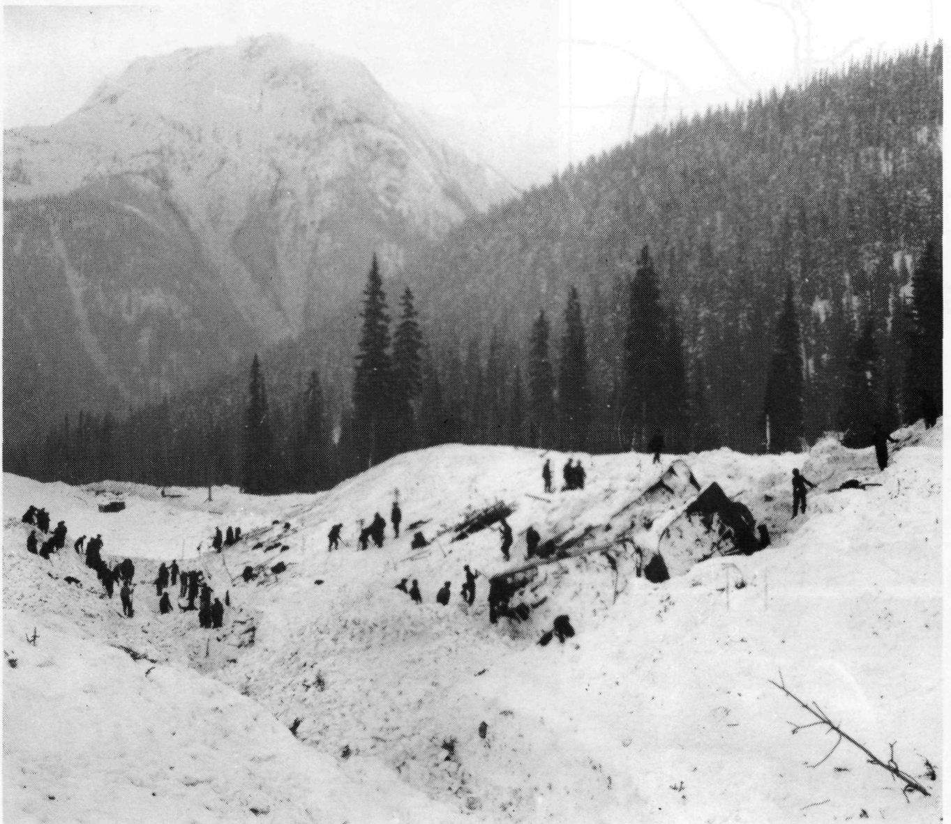
Figure 8: 1910 Disaster at 17 Shed
